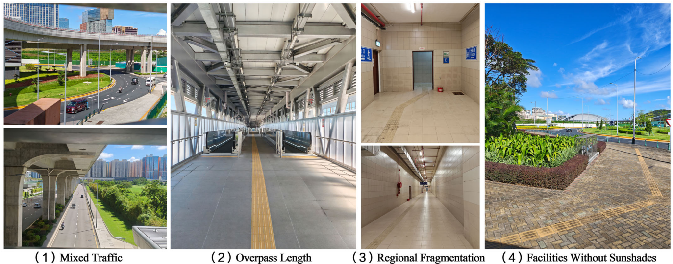
Figure 2. Current situation and problems at Macau LRT Union Hospital Station. (1) Mixed Traffic. (2) Overpass Length. (3) Regional Fragmentation. (4) Facilities Without Sunshades. (Image source: Photographed by the author).
